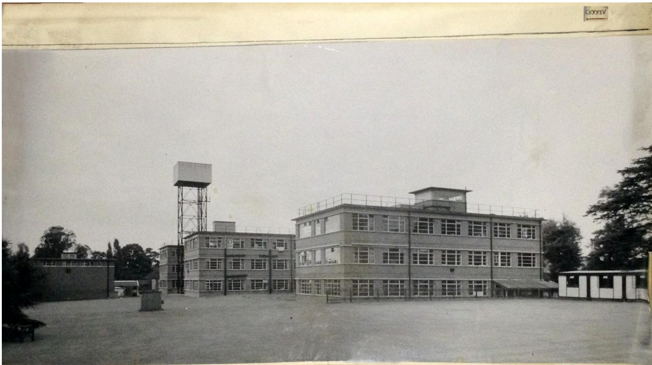
View of The Laboratories from the North East
