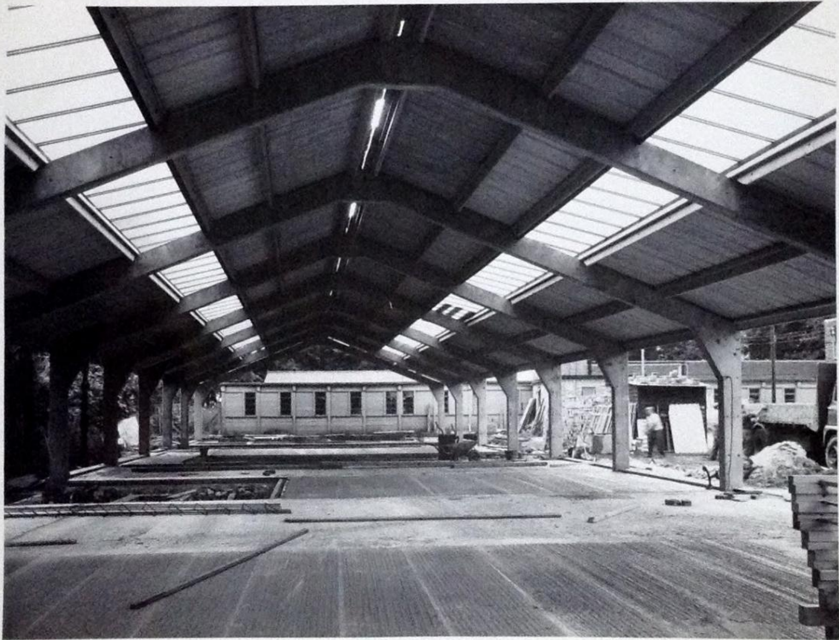
PREPARING THE NEW (CRFEP) LAB. FOR THE 1963 "OPEN DAYS".
