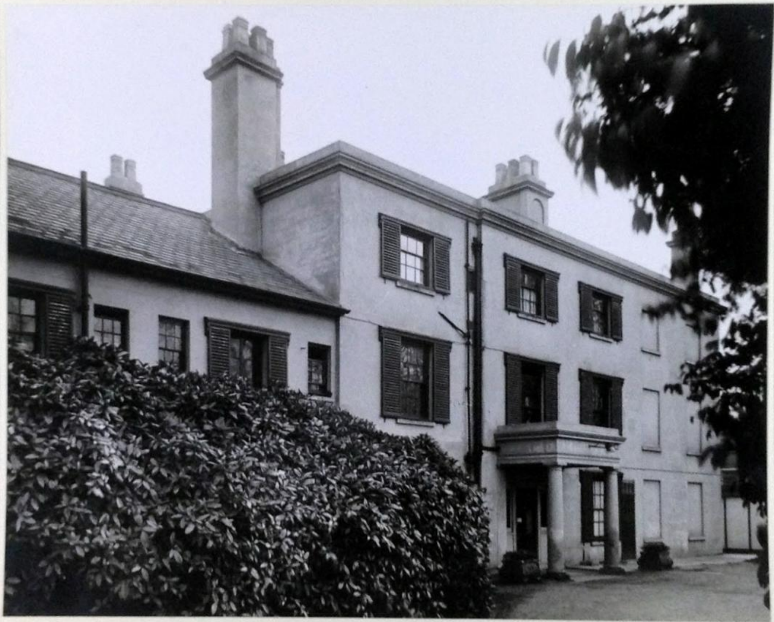
HAREFIELD HOUSE - from the North-West
