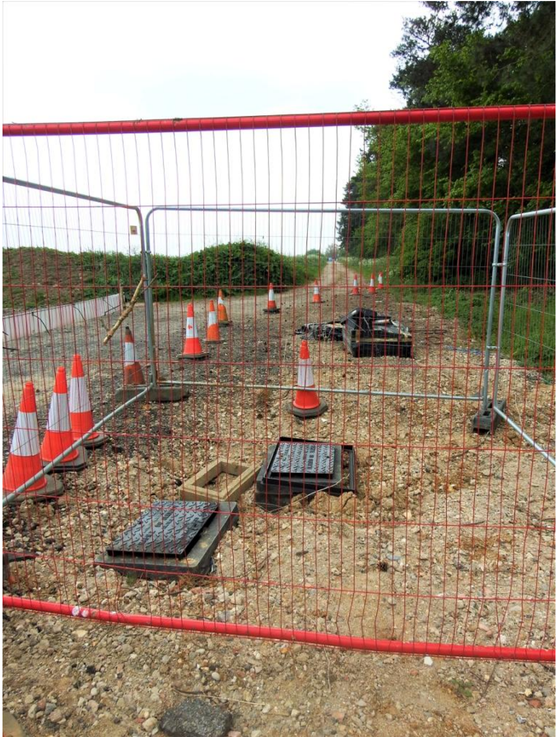
Photograph 25. New manhole covers.
