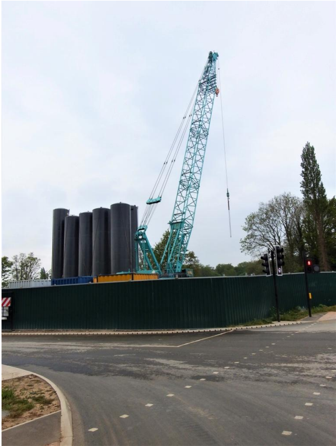
Photograph 26. Pile driving by Moorhall Road.
